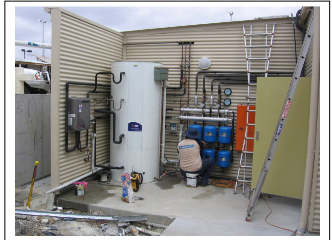
Installing the hot water tank, pumps, controller, booster and other components
